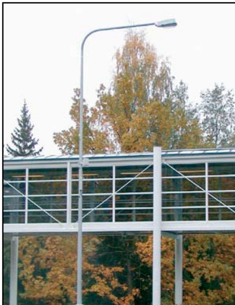
Base station integrated into lightpole
