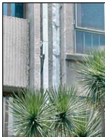
Base station blended into building facade
