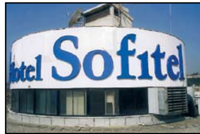
Base station blended into building facade
